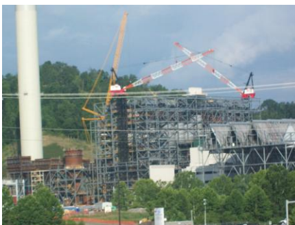
Dominion Coal Energy Plant
