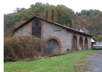
Clinchfield Steam Building
