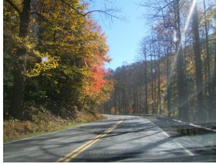
View on Hwy 83 in Dickenson County
