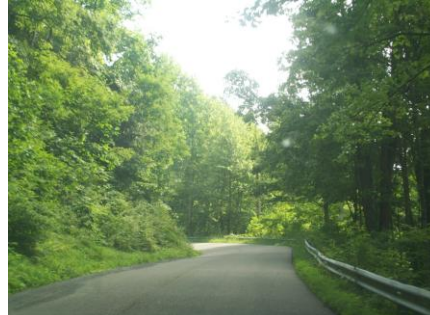
View on Hwy 380 in Buchanan County
