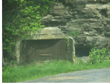
Splashdam #6 Mine Site
