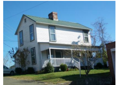
Railroad Section Manager's Home
