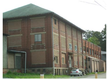
Freight Depot in Appalachia
