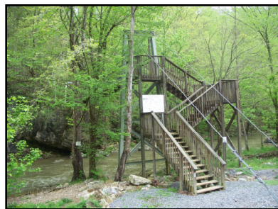
Suspension Bridge across Clinch River
