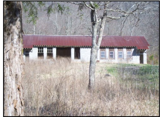
Potential to convert old school into lodging facility for ATV riders if building is still structurally sound.
