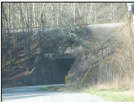
Tunnel one passes through as one nears Hagan ATV Trailhead.
