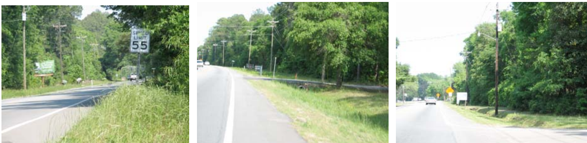
Utility wires along the proposed route of Bluffton Scenic Byway take away from view shed.
