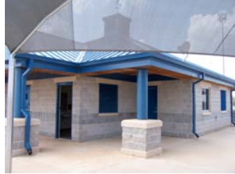
Recessed shelter area
