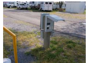
Double electric pole
