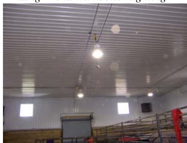
Retractable ceiling electrical outlets
