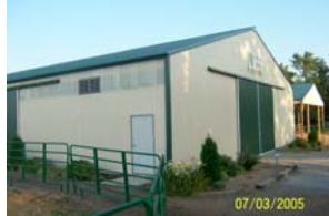
Enclosed Barn (existing)
