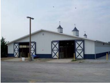
Existing Stables next to Arena
