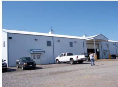
Arena Complex - Entrance on side
