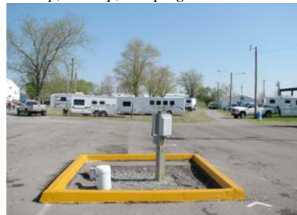
Electric/Water hookups on asphalt (Try to avoid this)
