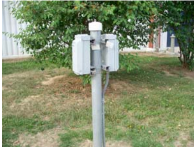
Electrical hook-ups and water for rigs
