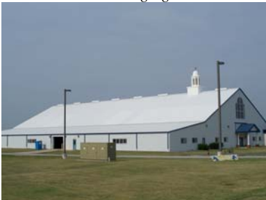
White roof works best. NO skylights
