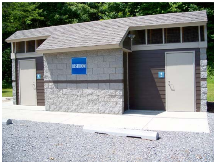
Public restroom facilities for elk viewers and other visitors to the area.
