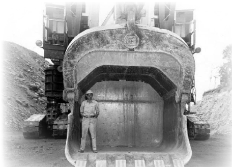
Big Shovel - Greenville
