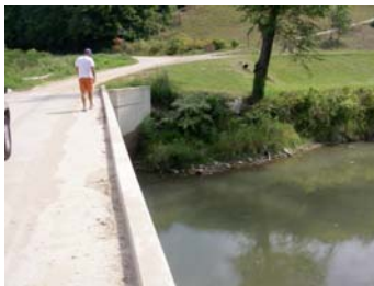
At Noble Landing Bridge on Troublesome Creek
