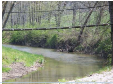
Multiple swing bridges
