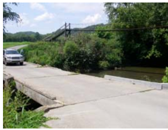
Round Bottom Access Bridge on Quicksand Creek
