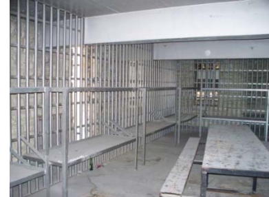
Interior view of the large interior cell
