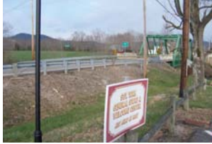
Bridge crossing Wolf River
