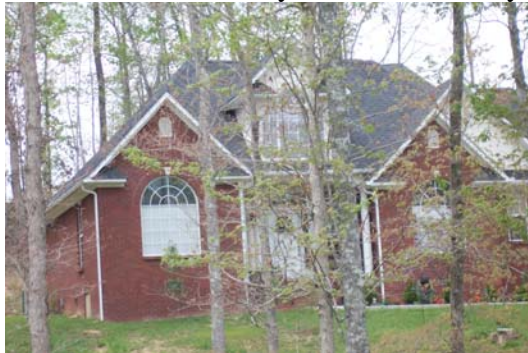
(Apple Creek Subdivision being built – Nice homes)
