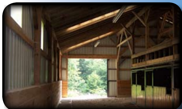
Natural side and overhead lighting
