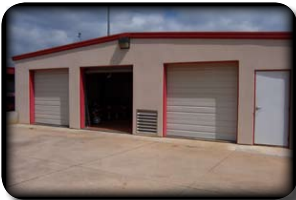
Equipment facility in Alpharetta Georgia
