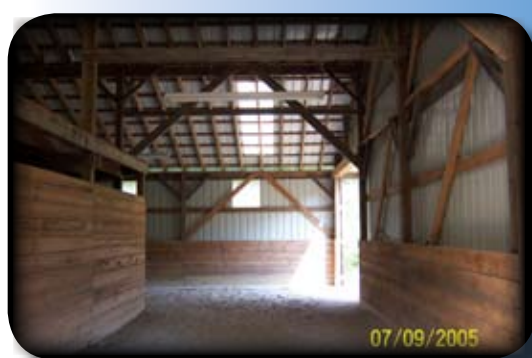
End of arena has two double sliding doors.
