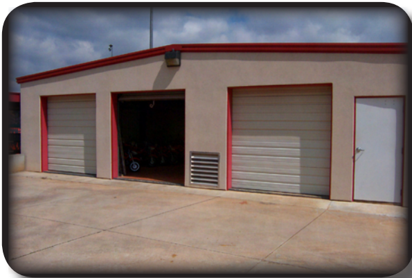
Equipment facility in Alpharetta Georgia
