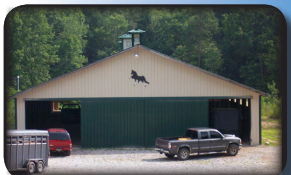
Front of building has double sliding doors.
