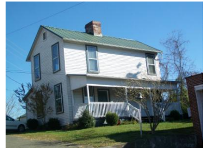
Railroad Section Manager's Home
