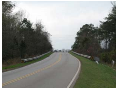
Bridge over abandoned railroad*
