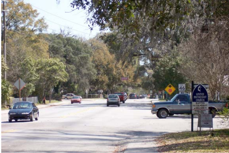
Intersection of SC 46 and Calhoun Street
