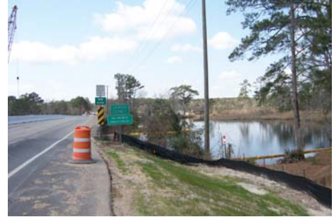
Bridge over New River
