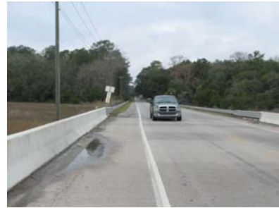
Stoney Creek Bridge
