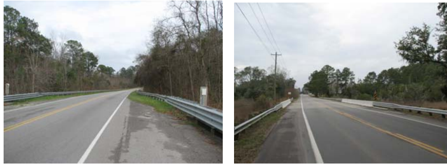
Metal DOT issued guardrails are functional yet not aesthetically appealing not eco-friendly.
