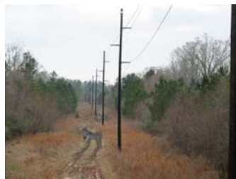
Railroad (Future Rails to Trails)
