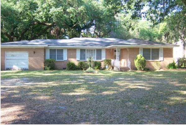
One of the homes located right on SC 46
