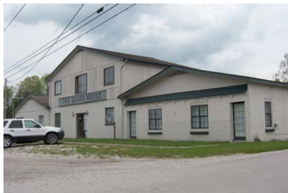
The main structure as it now appears
